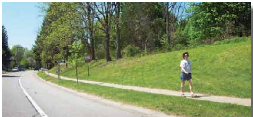
A long expanse of sidewalk along Palmyra Road provides an important connection to the village from surrounding neighborhoods.
