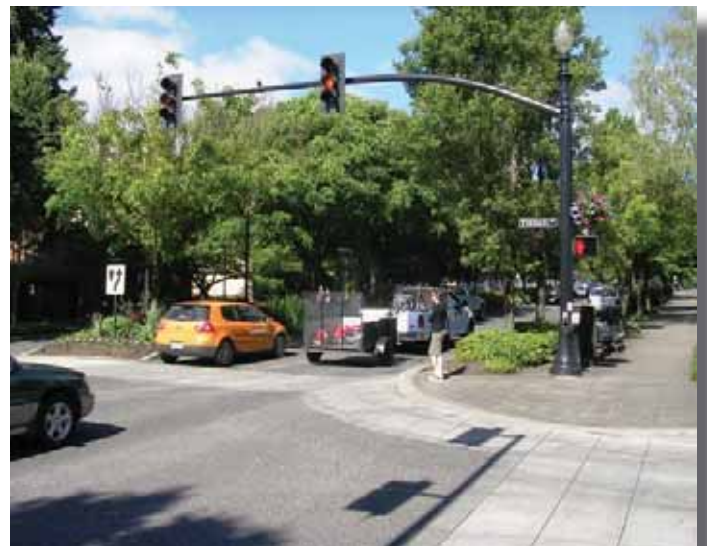
This street utilizes several design elements that help to make a safe place for both cars and pedestrians. Trees and planted medians help to enclose the street and encourage slow driving; curb bulb outs decrease the crossing distance for pedestrians; and clearly marked crosswalks alert drivers to stop for pedestrians.
