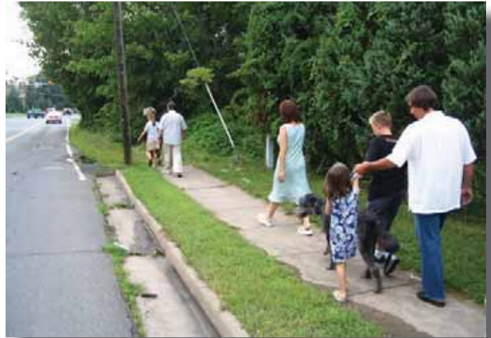
Inconsistent sidewalks and road design can be frustrating and unsafe for pedestrians, as this example from another community demonstrates.
