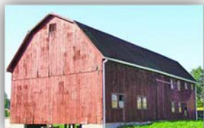
99 Willard Road Gambrel roof w/ basement Williams-Knickerbocker Built late 1800's
