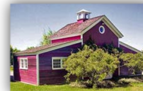
1 Mendon Center Road Gable roof - Reproduction Lusk Family Built 1999
