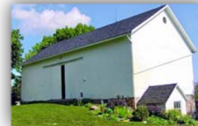
651 Mendon Road Gable roof Pugsley-Goodenough Built early 1800's
