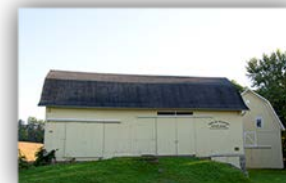
164 West Jefferson Gambrel roof Zornow-Schuyler barn Built late 1800's
